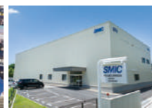
Chubu Segment Seto Factory
